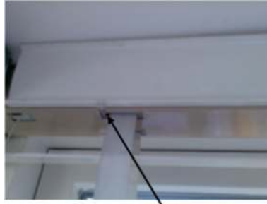
In many cases there are 2 plastic clips which hide the metal supports. Prise open carefully to allow the cover to drop free
