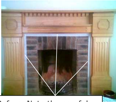
Before. Note the careful masking of the brickwork!
