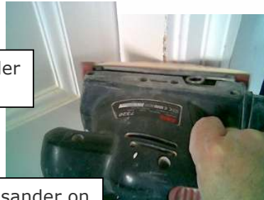
Using an orbital sander on door frame
