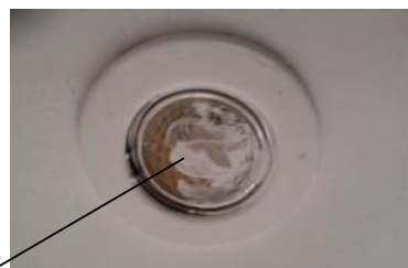
This is the result if you can't be bothered to mask off! (and this was done by somebody being paid to do it!)
