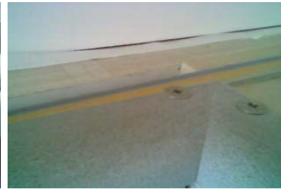
Masking over top of kitchen units
