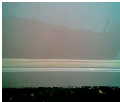
Masking applied to top of skirting board
