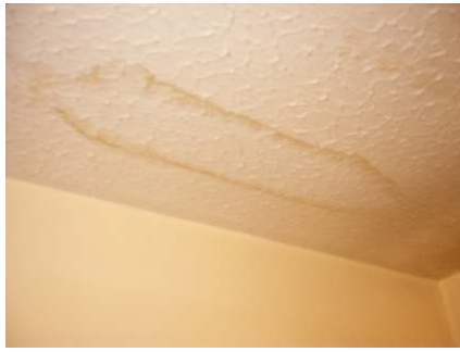
Water-damaged ceiling
