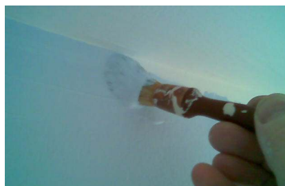
Cutting-in at the join between ceiling and wall using a sash brush
