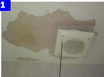
Unscrew the fan from the ceiling if possible
