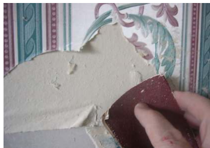
Sand torn paper back to sound surface
