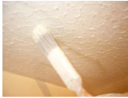
Apply stain block. Allow to dry. Paint with ceiling emulsion as normal
