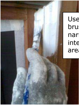
Applied Zinsser Allcoat Multi Surface Primer & Finish
