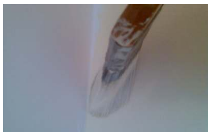
Cutting in at the join between two walls using a synthetic brush
